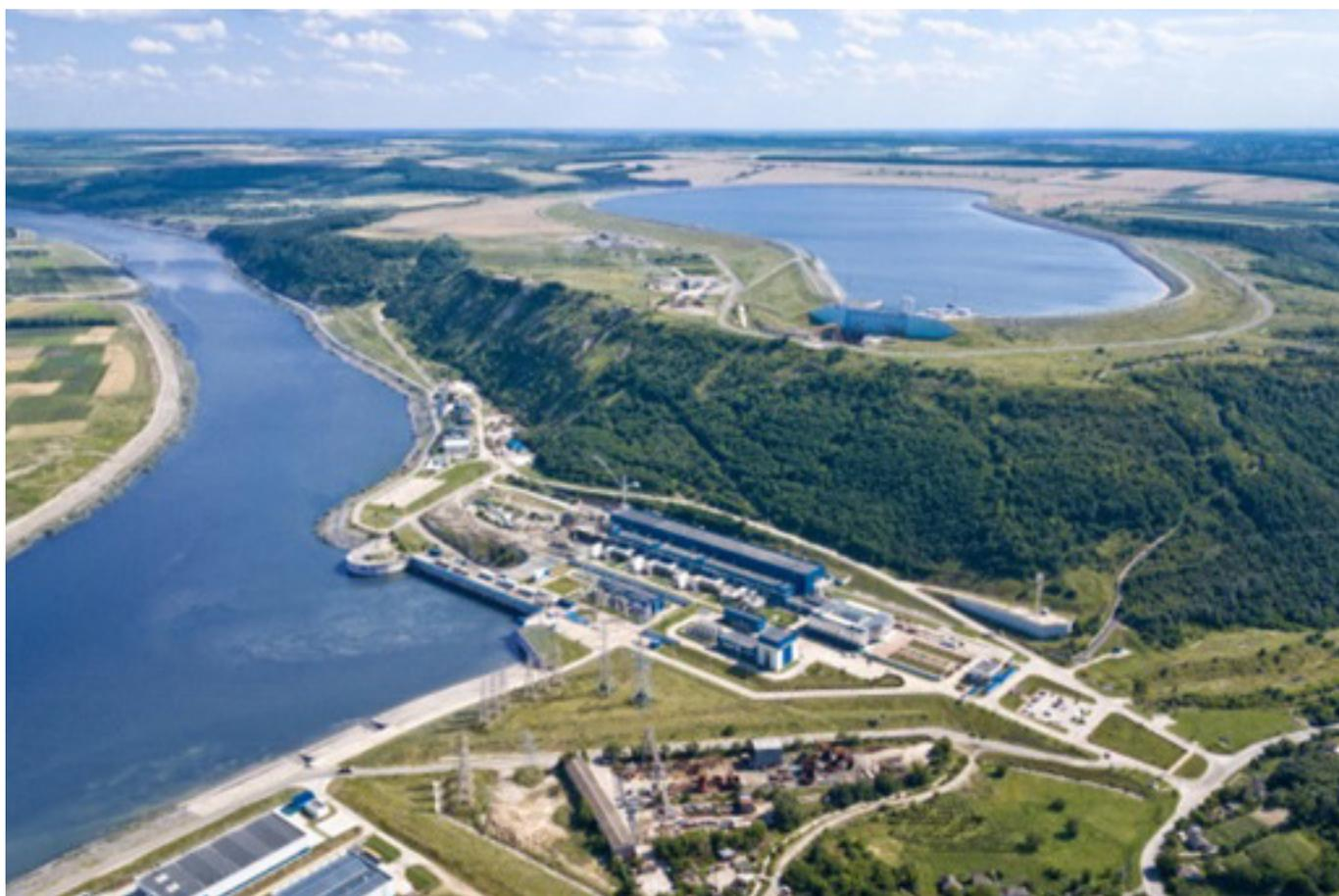
**Figure 1.5.** PSHPP with the largest reservoir built on the karst bank of the Dniester near Ocnita town; the reservoir is fed from the Dniester river.
